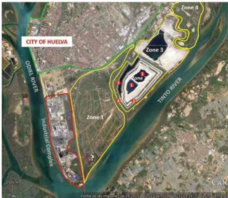
Figure 2. Aerial photograph of the area of the Tinto river marshes. (1) Settling ponds, dumping area of FY; (2) regulating reservoir, (3) perimeter channel, and (4) pumping station.
