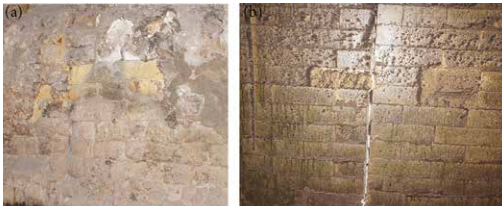
Figure 15. View of lining made of not alkali resistance fire clay bricks after 6 months of boiler operation (a) and made of alkali resistance fire clay bricks after 8 months of boiler operation (b).
