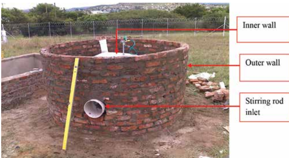
Figure 7. Constructed second wall of the biogas digester.
