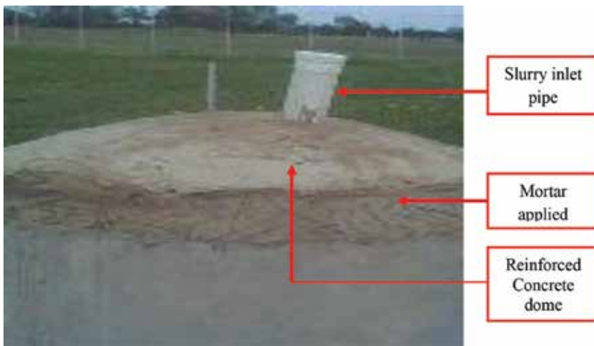
Figure 6. Biogas digester with a reinforced concrete dome.
