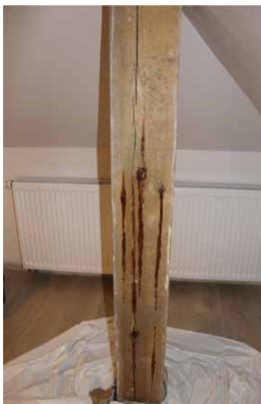
Figure 10. Resin melting in pine wood after exposure to microwaves radiated in practice by the 0.6 kW SAURUS device made in Italy (photo by CARSEKT).
