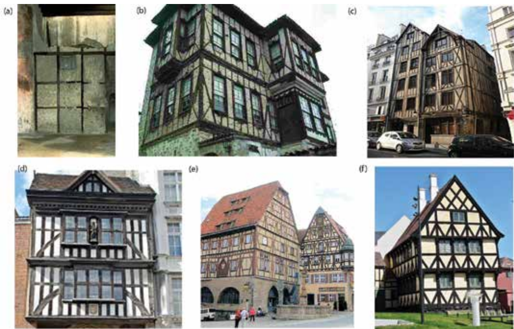
Figure 4. Historical timber-framed masonry buildings: (a) house wall from Herculaneum (opus craticium attested by Vitruvius in the first century BC); (b) nineteenth-century Ottoman house; (c) sixteenth-century timber-frame house in Paris (France); (d) St. Bartholomew's Gatehouse built in London in 1595 and survived to the 1665 great fire; (e) German typical timber-framed houses (Fachwerkhäuser); (f) Anne Hvide's House built in 1560, Denmark.
