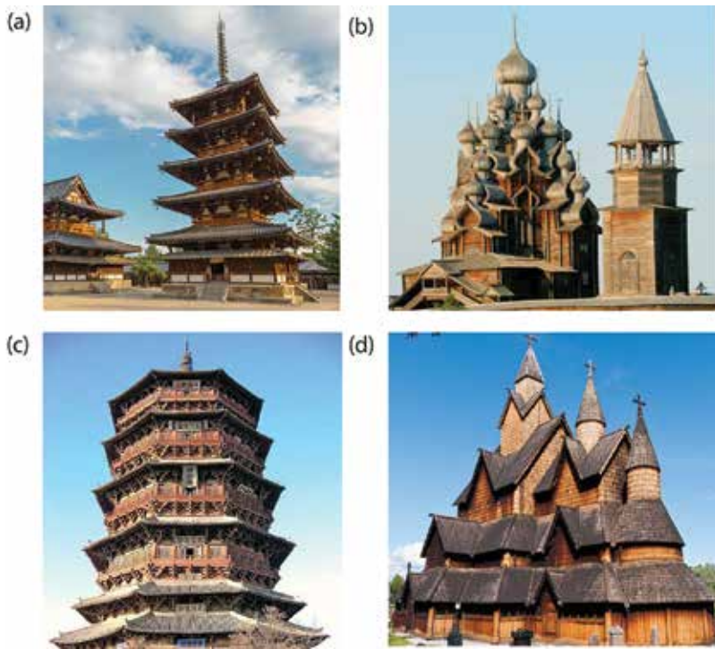
Figure 5. Ancient wood constructions: (a) Hōryū-ji Pagoda (Japan, 607 A.C.); (b) Kizhi Pogost Church (Russia, seventeenth century); (c) Fogong Temple Pagoda (China, 1056 AC); (d) Heddal stave church (Norway, thirteenth century).
