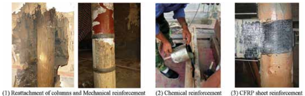
Figure 10. Reinforcement techniques of ancient wooden buildings.
