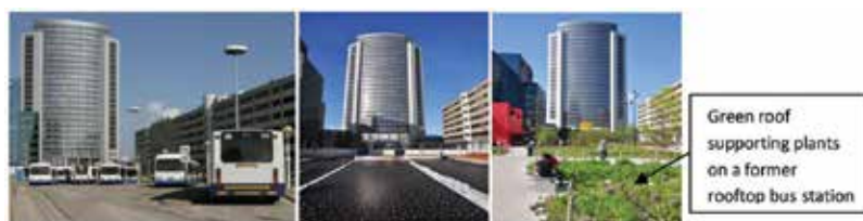
Figure 3. The roof park built on the former Orlyplein Bus Station deck , before, during and after construction.
