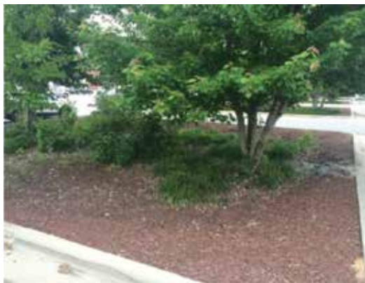
Figure 5. A bioretention cell with trees and shrubs in Raleigh, North Carolina, USA.
