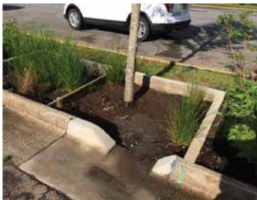
Figure 6. A tree pit receiving urban sediment from an adjacent parking area, Greensborough, North Carolina, USA.
