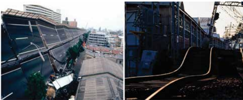
Figure 2. A damaged massive bridge and railways by Kobe EQ, 1995, January 17, M7.3.
