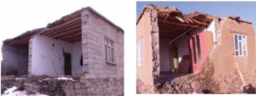
Figure 21. Out-of-plane mechanism of the brick buildings [42].
