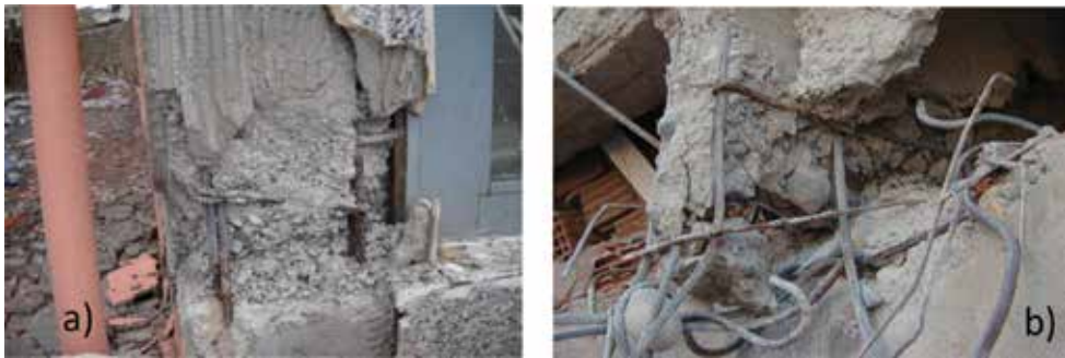
Figure 17. Failure of column due to poor concrete quality during: (a) Van earthquake and (b) Bingöl earthquake.
