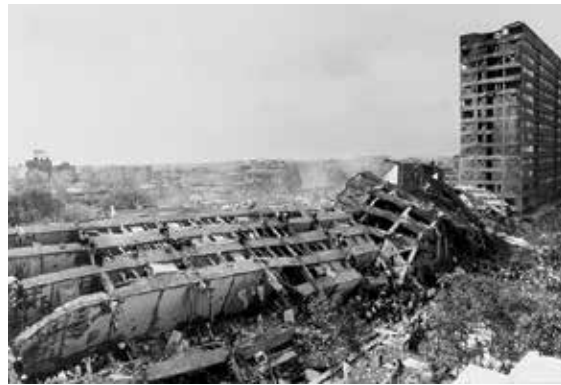
Figure 4. Collapse of the Nuevo Leon buildings (south building remained standing at the far side, picture by Marco Antonio Cruz).
