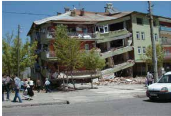
Figure 14. Collapse of adjacent buildings during the Bingöl earthquake.
