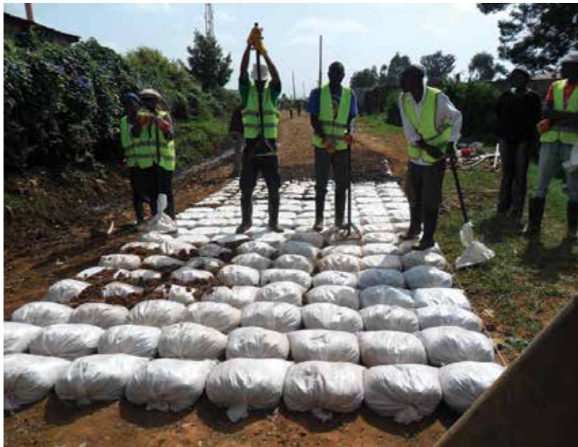
Figure 6. Practical manual compaction method for community work.
