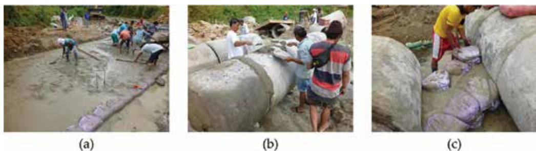
Figure 19. Work items managed by the community: (a) Leveling the concrete surface; (b) filling the gaps of RC pipes; (c) laying Do-nou.
