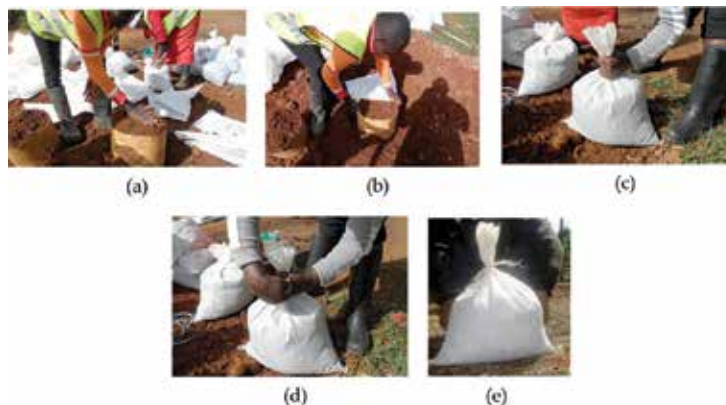
Figure 9. Procedures for filling the Do-nou bags with granular material: (a) Measurement container; (b) transferring material to bag; (c) open end of the bags above the fist; (d) tying with nylon string; (e) Do-nou filled with granular material.
