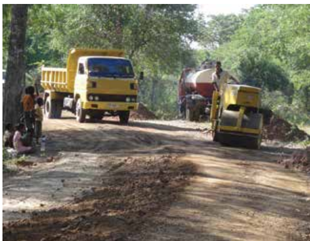
Figure 3. Road rehabilitation work in Timor Leste, using the equipment required for LBT.
