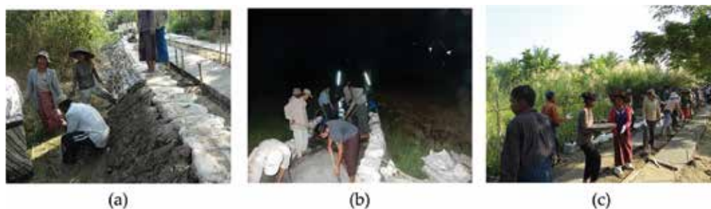
Figure 15. Construction at village K: (a) Covering Do-nou with clay; (b) working at night; (c) bucket brigade for casting concrete.
