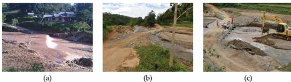
Figure 20. Vented ford affected by a typhoon and emergency work done by the provincial government: (a) Overflowing; (b) deposited sedimentation; (c) removing the sedimentation by the excavator of the provincial government for emergency.
