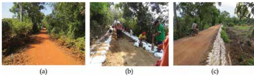
Figure 12. Construction of road embankment with Do-nou retaining wall: (a) Before construction; (b) construction of the embankment with Do-nou retaining wall; (c) after construction.
