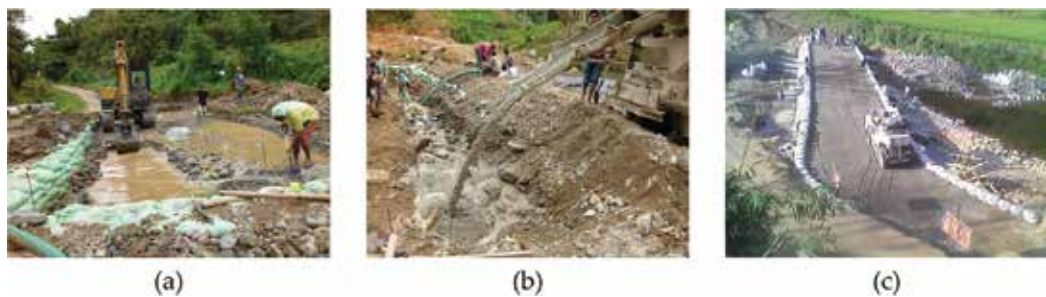
Figure 18. Work items managed using equipment provided by local government: (a) Excavation of the cut-off-wall and foundation; (b) transit mixers and water pump during casting concrete; (c) compaction of base course with roller.
