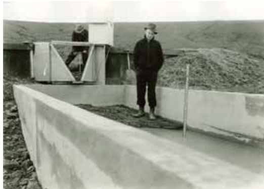
Figure 10. H flume and downstream sediment trough that catches all sediment from the bare, steep watershed after an extreme event.
