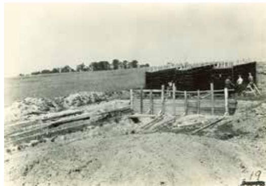
Figure 8. Construction and installation of three lysimeters at the NAEW.
