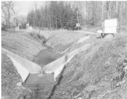
Figure 6. Short-crested V-notch weir replaced the Parshall flume upstream in the view on a larger NAEW watershed.
