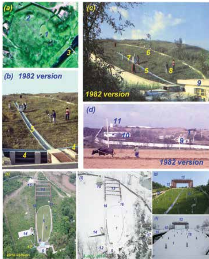
Figure 12. Finalization of the artificial catchment Hydrohill, its previous version (1982–1995) and renovation version (since 2012). (a) a satellite image showing Hydrohill and the whole hillslope area to be excavated of ca 4700 m 2 ; (b) and (c) the previous version of equipped Hydrohill; (d) the environment of Hydrohill. 1-land surface of Hydrohill; 2-an uncompleted artificial catchment; 3-the outlet of the Bloomhill Basin showing a discharge measuring structure of the gauging station; 4-the side trench perpendicular to the main trench at the watershed outlet; 5-the main longitudinal trench with layered troughs; 6-energy budget monitoring apparatus; 7-a scanning recorder for soil water potential from distributed sensors; 8-the neutron moisture gauge is in operation; 9-underground house for the discharge measuring structures; 10-laboratory for the calibration of neutron moisture gauge (1982–1988); 11-water supply tower; 12-two lysimeters with layered runoff troughs, 4 × 8 m 2 each, two different soils; 13-movable rainfall simulator at rest; 14-a reservoir for water supply of rainfall simulator; 15-a dual polarization Doppler precipitation radar for the areal precipitation monitoring of the Bloomhill Basin with drainage area of 80 km 2 ; 16-tracks for the moving of rainfall simulator; 17-laboratory for instrument measuring of isotopes; 18-various monitoring wells, sensors, samplers.
