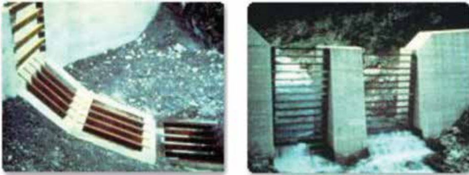
Figure 18. The debris flow dehydration.
