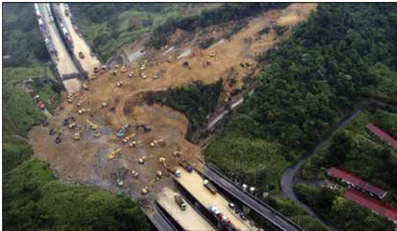
Figure 12. Landslide after rain in 2010, Taiwan.
