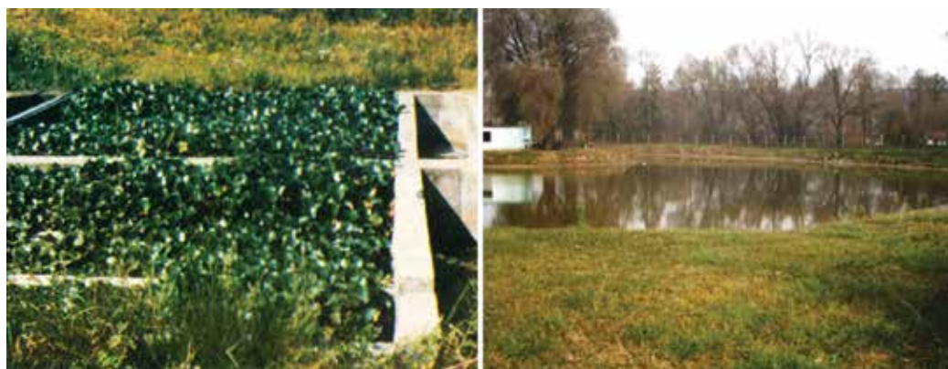
Figure 7. Basin for sanitary hydrophytocultures and basin for sanitary aquacultures on the WWTP Sokobanja.
