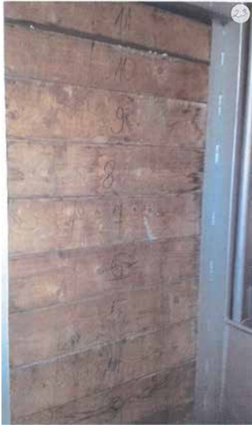
Figure 4. The plank barrier seen from the lashing equipment room. Wood pellets in the cargo hold are visible between planks 10 and 11. The barrier is evidently not gastight. (CORINA). Source: Police photo file #23 [8].
