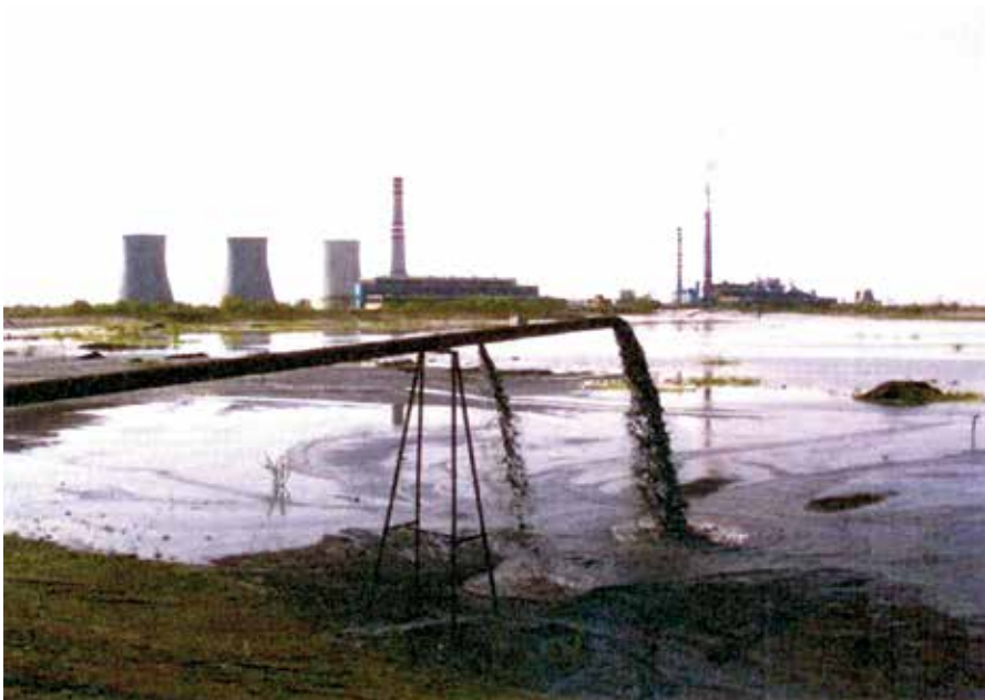
Figure 4. Filling tailing pond.
