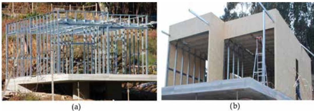
Figure 1. Example of a low-rise LSF residential building at construction stage [14]. (a) Steel frame; (b) OSB external layer.
