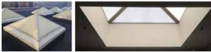
Figure 6. Existing skylights from the outside and from the inside.
