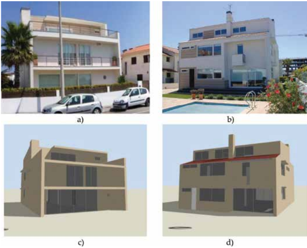
Figure 18. LSF residential building and DesignBuilder model [9]. (a) Front view. (b) Rear view. (c) Front view. (d) Rear view.
