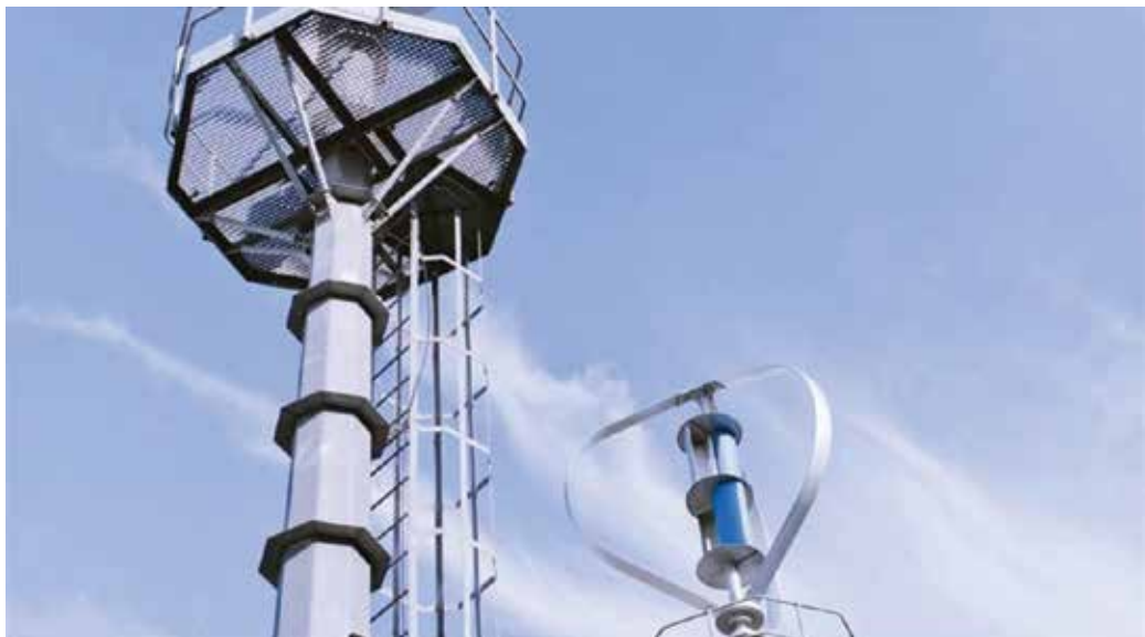
Figure 3. Huebner-Giessen 3 kW wind turbine here.
