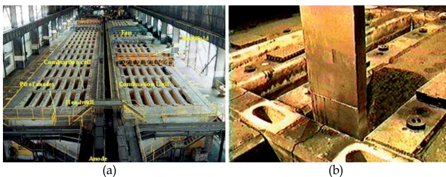
Fig. 1. a) Anode baking furnace building overview; b) Petroleum coke being unpacked from anode coverage by vacuum suction.
