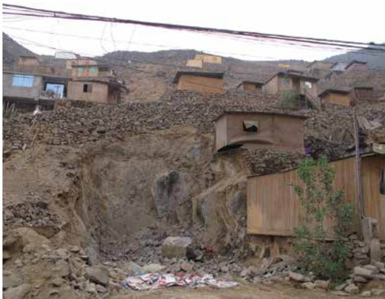
Figure 6. As people flatten the plots to then build their house, they contribute to the instability of the slope and increase the risk for others. Source: Photo by Rita Lambert.
