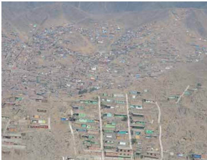
Figure 8. The vertical staircases of JCM are planned and built in such a way that they increasing the risk of accidental falls. Source: Photo by Rita Lambert.
