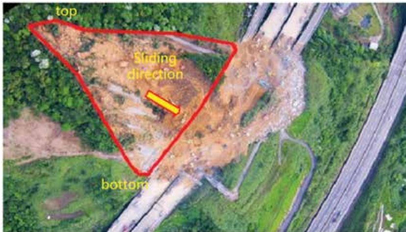
Figure 9. Side boundaries of the landslide and the freeway limits [23].
