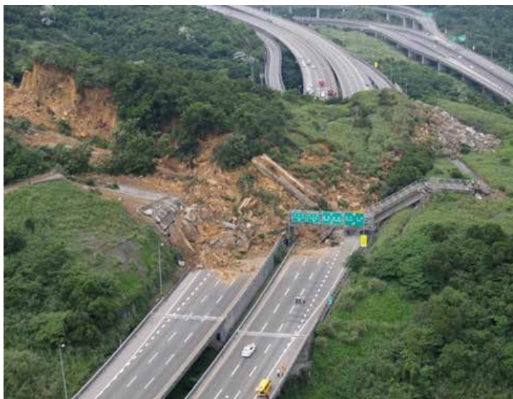
Figure 3. Photograph of the landslide at Freeway No.3 (Source: http://www.nasc.gov.tw/files/duty_news_files/_4251883.JPG ).
