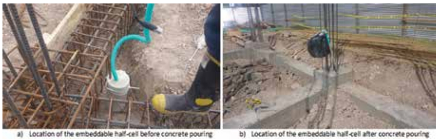
Figure 9. Installation of the embeddable half-cell.
