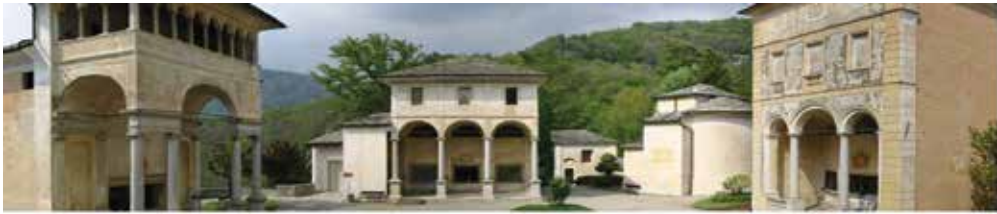
Figure 11. Overall view of the square of the courts.
