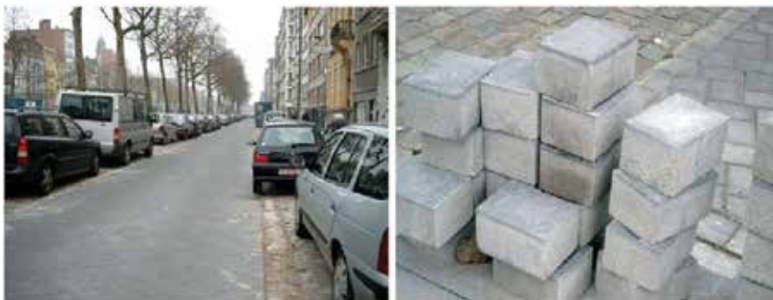
Figure 4. Separate parking lanes at the Leien of Antwerp with photocatalytic pavement blocks [15].
