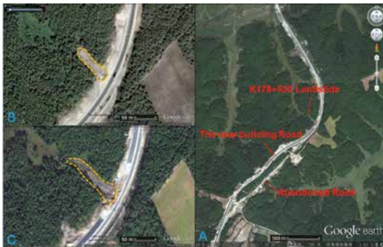
Figure 5. Satellite photos of K176 + 500–K179 + 900 section of Bei'an-Heihe Highway (Google earth). (A) Landslide in K178 + 530 section (in 2000); (B) satellite photos of K178 + 530 (2004.6); and (C) satellite photos of K178 + 530 (2010.9).
