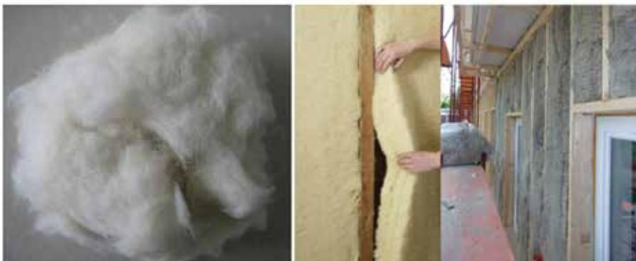
Figure 11. Sheep wool and its application in building construction [9].
