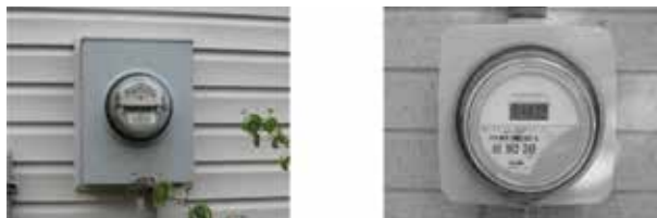
Figure 2. A typical residential analog and digital (smart) electric meter with a digital display showing cumulative kilowatt hours used.
