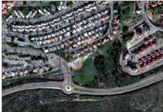
Figure 8. The experimental site is located at the western end of the sewage line adjacent to HaAtsmaut Street (blue rectangle). It includes 12-in. diameter iron pipes carrying on the order of 1000–1200 m 3 sewage water per day, and an average 100 m 3 /h during peak flow.
