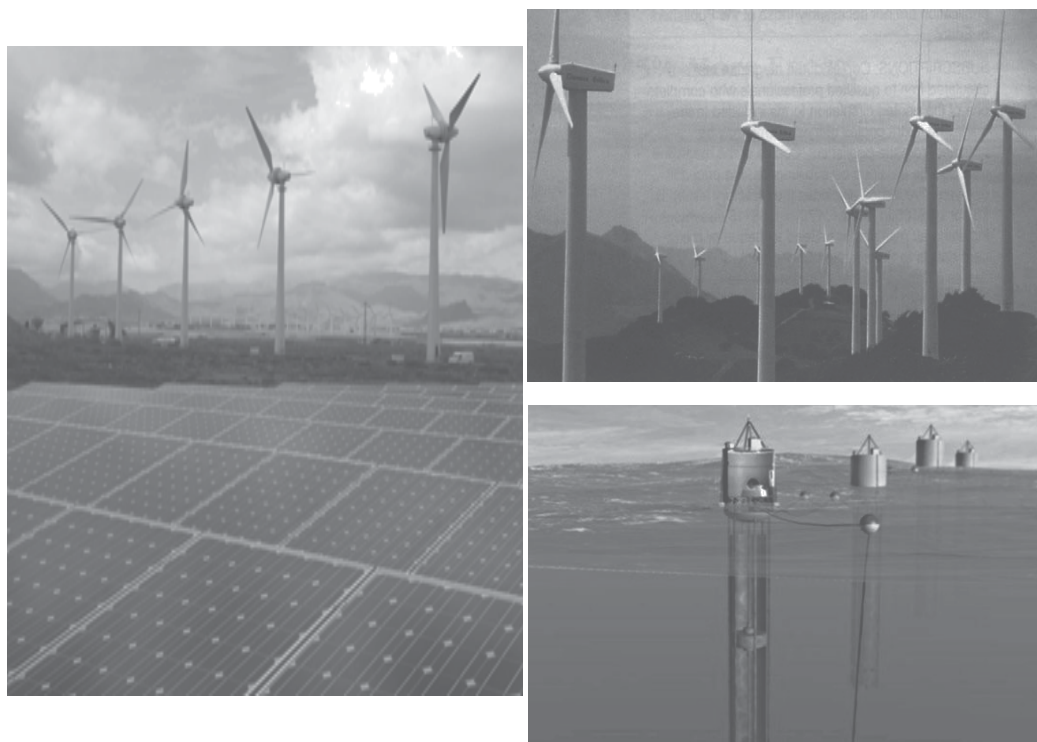
Fig. 4a (Upper Left) Wind Farm (Kalogiros, 2005); 4b (Right) Wind turbines and PV cells of Sureste SWRO plant (Sadhvani, 2008; IDA Conference, 2008); 4c (Lower Left) Wave Energy. The Aquabuoys 2.0 is a large 3 meter wide buoy tied to a 70-foot-long shaft. By bobbing up and down, the water is rushed into an acceleration tube, which in turn causes a piston to move. This moving of the piston causes a steel reinforced rubber hose to stretch, making it act as a pump. The water is then pumped into a turbine which in turn powers a generator. The electricity generated is brought to shore via a standard submarine cable. The system is modular, which means that it can be expanded as necessary (Chapa, 2007).
