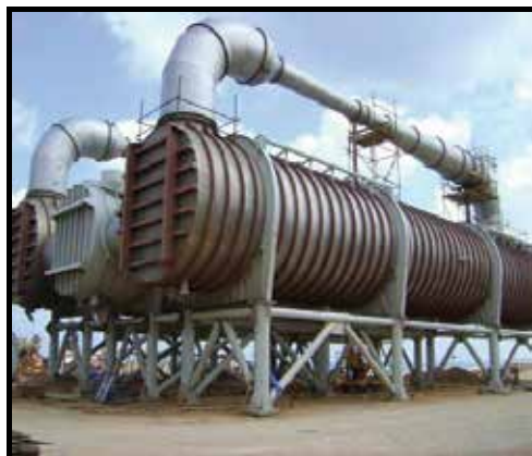
(a) Circular vessel evaporator.
