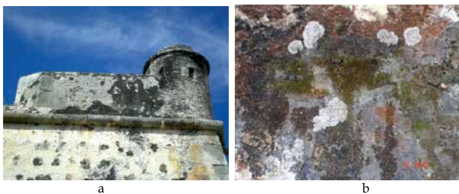
Fig. 11. Aspect of the biodeterioration in the historic buildings of San Francisco de Campeche City. (a) Fort San Carlos. (b). Microbial community at West wall of Fort San Pedro.
