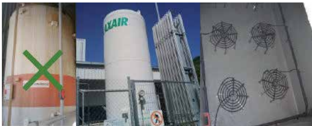
Figure 15. Dosing system for sewage.
