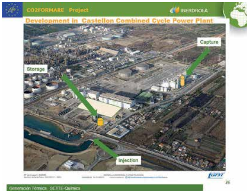
Figure 23. Castellón Power Plant. Courtesy: Iberdrola.
