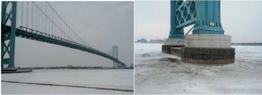
Figure 1. The ice cover around bridge piers (Ambassador Bridge, Windsor, ON, Canada, 2015)
