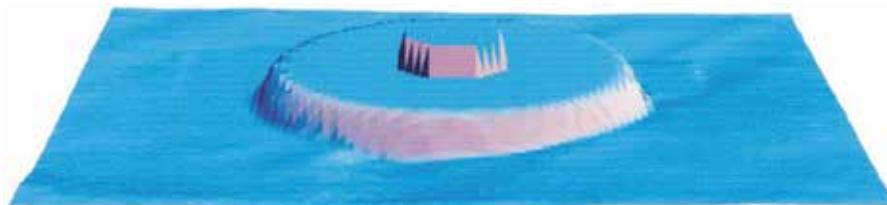
Figure 1. Submerged dissipation platform to protect the Bugio lighthouse, situated at the mouth of the Tagus estuary.
