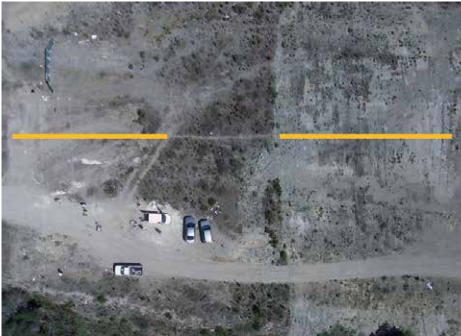
Figure 5. Lakatameia underground pipeline as observed from UAV
