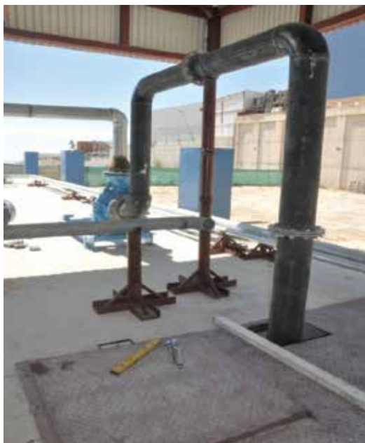
Figure 8. Pipe network during construction
