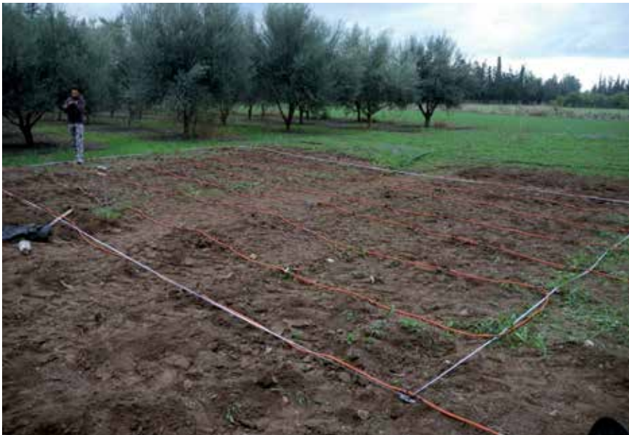
Figure 1. Area of interest. A pipeline was buried at a depth of approximately 1 meter.
