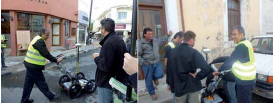
Figure 2. Geo-radar Scanning of the Paphos water utility network
