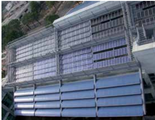
Figure 4. Final Photo of experimental installations in test filed
