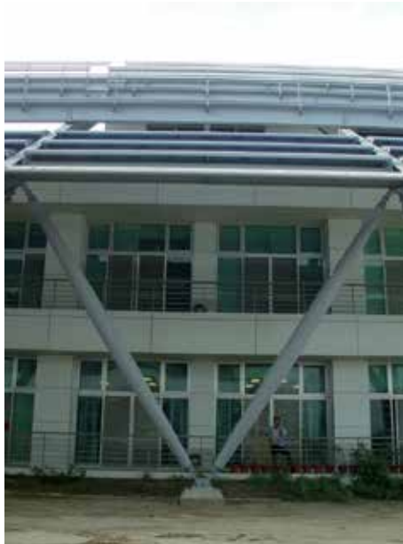
Figure 5. Final Photo of experimental installations with Integrated Photovoltaic and Sunshading Board
