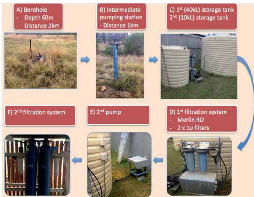
Figure 12. An Example of a rural home water treatment setup: (A) The borehole is approximately 2 km from the patient's residence and is determined by the geology of the area. (B) An intermediate pumping station operated using air pressure. (C) Storage tanks are continually replenished from the bore to ensure an uninterrupted water supply. (D) A basic pre filtration cartridge filter (located in the silver casing) and two micron filters pre treat the water (E) A second pump located approximately 100m from the patients residence (F) A second set of micron filters and carbon tanks. This is located underneath the patients home and feeds directly to dialysis machine inside the bedroom.
