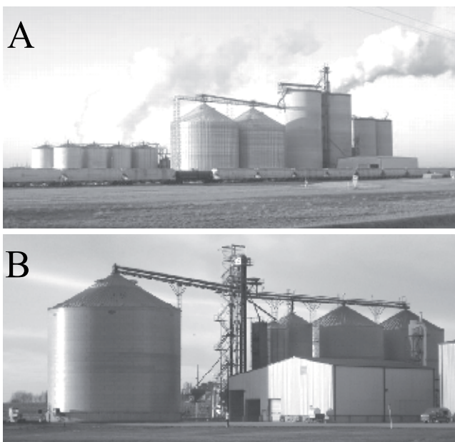
Figure 3. U.S. dry grind corn-to-ethanol manufacturing plants. A. 450 x 10 6 L/y plant. B. 80 x 10 6 L/y plant (Photos courtesy of Rosentrater).
