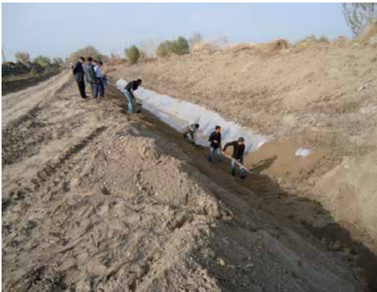
Figure 4. Covering of plastic with compacted soil
