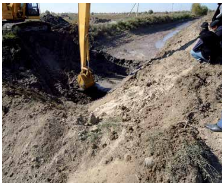
Figure 2. Cleaning the bottom and the banks of the channel
