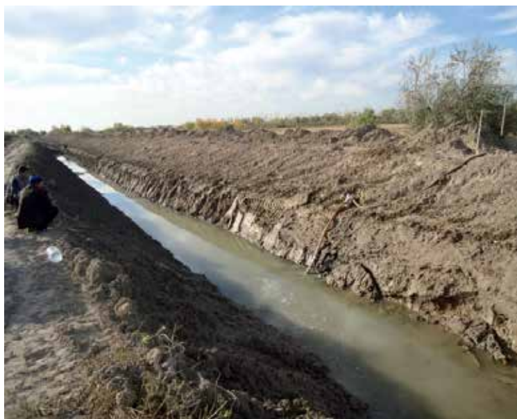
Figure 5. Gravity flow of water in the plastic lined channel
