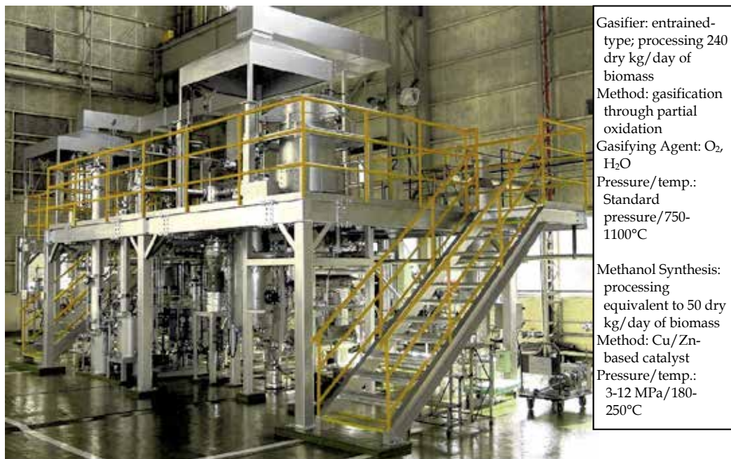
Fig. 8. "Norin Green No. 1", a test plant of gasification and biomethanol production, located in Nagasaki Research & Development Center, Mitsubishi Heavy Industries Ltd, Nagasaki, Japan.
