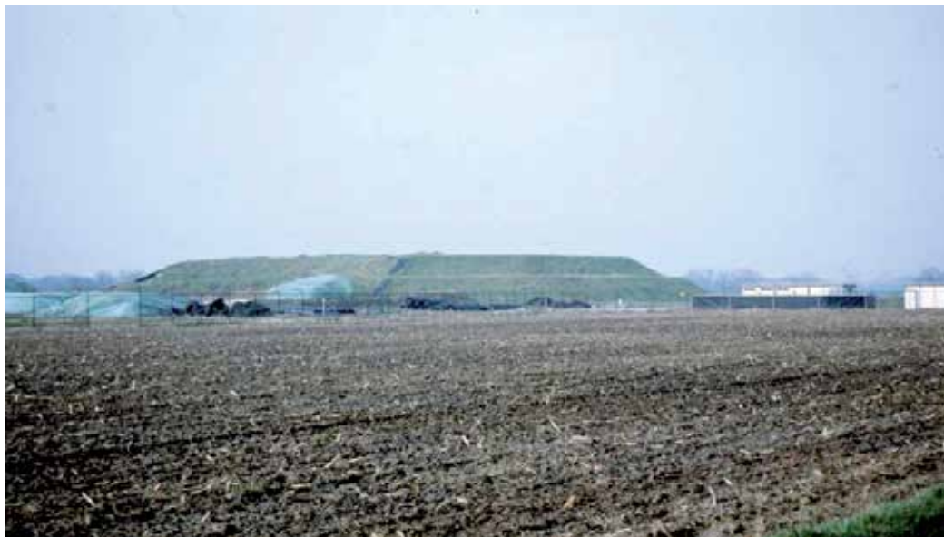
Photo from the mid-1990s of a temporary storage site for 200 000 tons of soil contaminated with waste HCH isomers.
