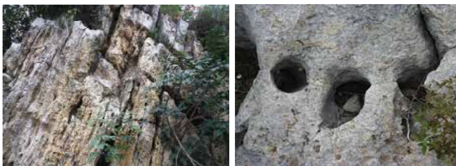
Corrosion on the surface of limestone
