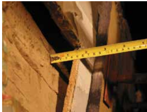
Fig. 2. Delaminated wall paintings in Eastern Audience Hall of Potala Palace
