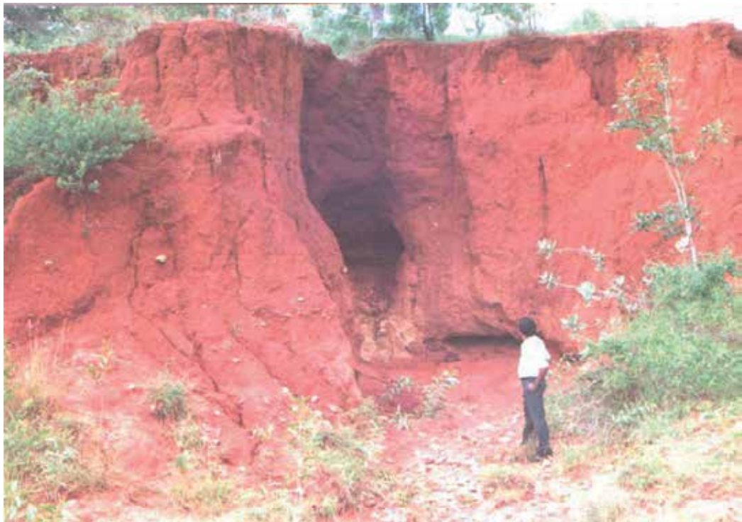
Fig. 9. Most catastrophic form of erosion: Gully erosion
