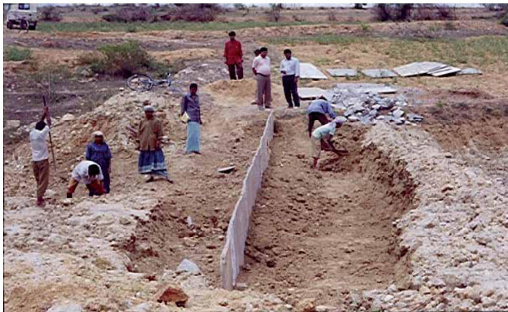
Fig. 17. Providing sub-surface drainage to manage soil salinity/alkalinity
