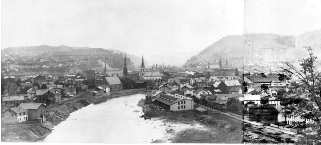
Fig. 2. Johnstown before the flood. View looks down Stoney Creek River toward the Stone Bridge. Note the infilling at the river banks and the construction virtually in the river bed. You can imagine that it would not take much of a flood to float these wood frame structures from their foundation can carry them off.
