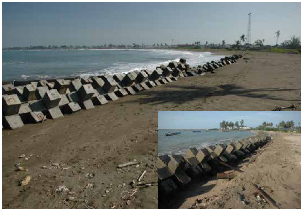
Fig. 8. Protective concrete structures set in place along (a) northern and (b) southern coasts of the Peninsula of Meulaboh. Note that only the southern coasts were actually eroding; along the northern coasts the beaches were accreting.
