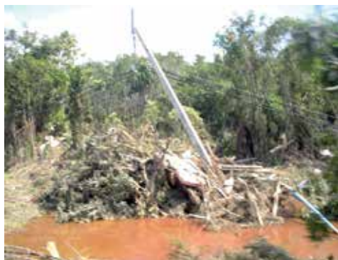
Photo 3. Electric pole tilted by collision with tsunami driftwood (Khao Lak, Thailand)
