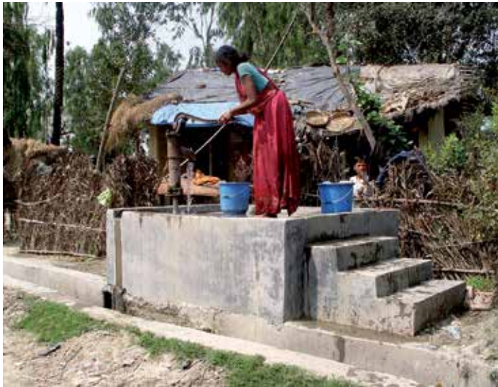
Fig. 5. Example of 'flood-proofed' water well (Photo: courtesy of Jørgen Kristensen, Danish Red Cross)
