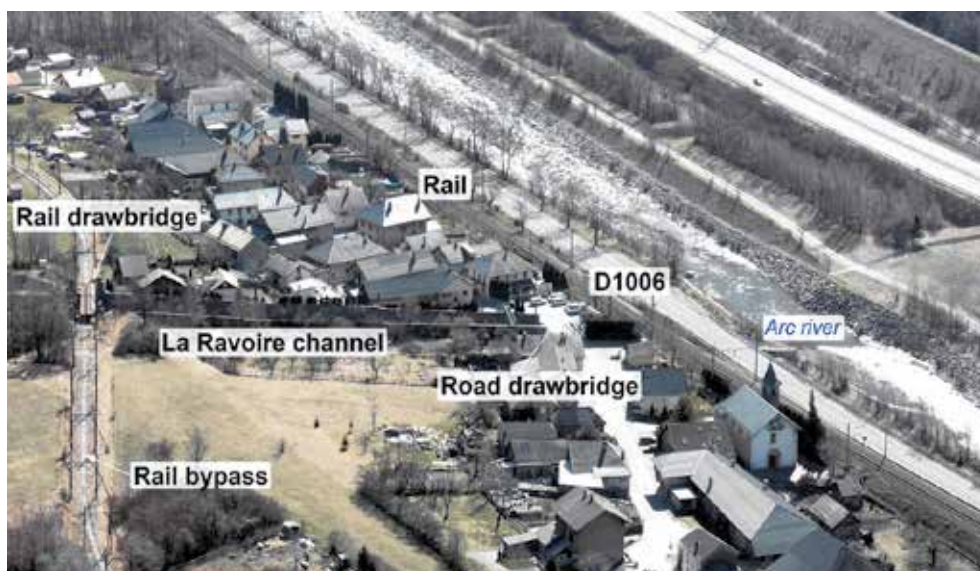
Fig. 8. View of Pontamafrey village constructed on the debris cone of La Ravoire. La Ravoire channel crosses the village the international line of high-speed train (TGV) which links Paris to Turin and the road way D1006.
