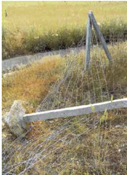
Photo 7. Old inappropriate fence destroyed by bears highway crossings
