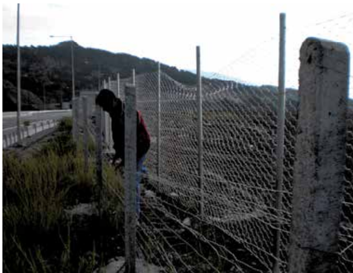
Photo 8. New fence permeability problems due to inadequate standards (missing of the upper bent part)
