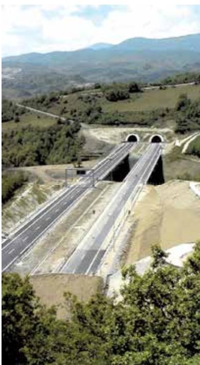
Photo 4. Partial view of the mitigated Egnatia Highway
