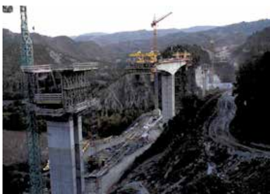
Photo 1., 2. and 3. Construction of the Egnatia highway
