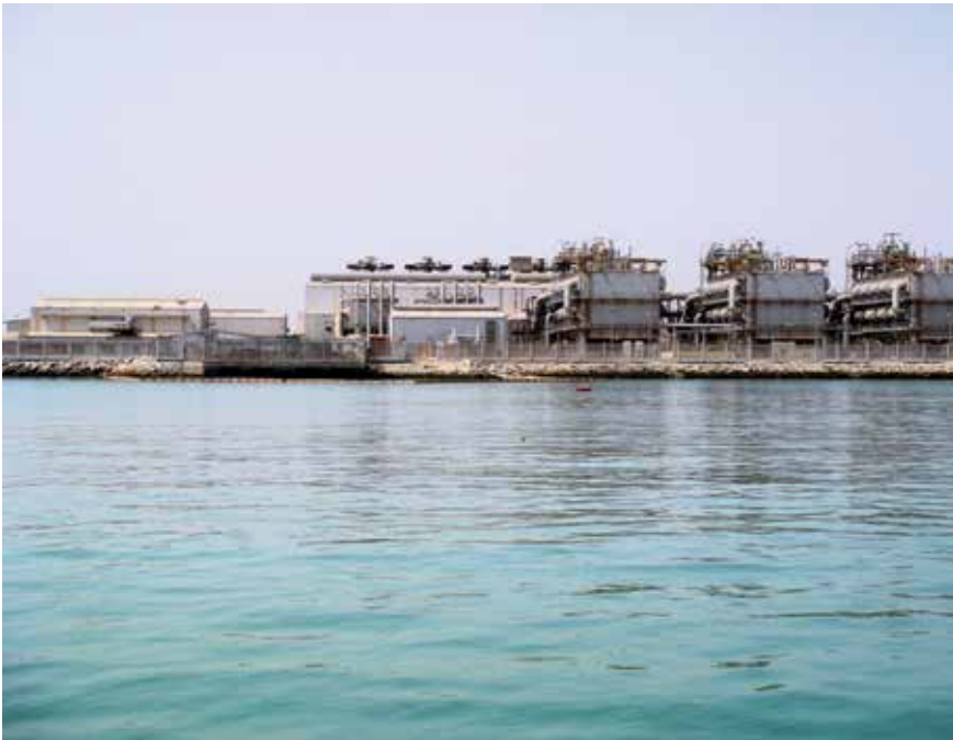
Figure 5. Marine organisms at the proximities of desalination plants are influenced by chemical, physical and thermal pollution. Reduced levels of diversity and abundance of macrobenthos were recorded adjacent the outlet of this MSF desalination plant along the eastern coastline of Bahrain (2012).
