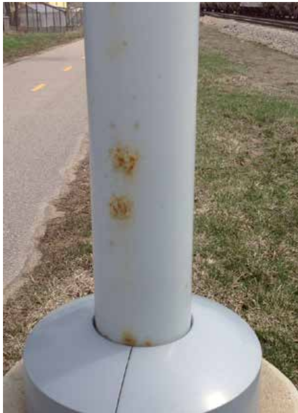
Figure 11. Corrosion underneath a coating failure. This lamp post was in service for less than 5 years before corrosion was visible at defects in the coating. SCALE: The lamp post is approximately 115 mm.
