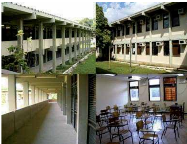
Fig. 1. Photograph of the building. In clockwise: external side with glass windows, classroom, corridor and external side with corridor along
