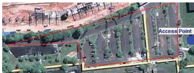
Fig. 4. Photograph of the parking lot
