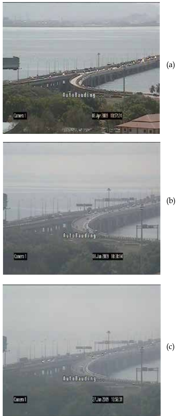
Fig. 7. Three photographs of Penang Bridge at different atmospheric aerosol concentration level
