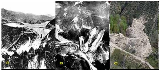
Fig. 3. Saint Dam Disaster. Francis, Francis, Los Angeles County, California, USA. Completed in 1926, the March 12, 1928, catastrophically failed due to geotechnical calculation errors during execution, killing more than 600 people. \_Francis\_ Dam Images from the start of the gap (A), after the disaster (B) and current image of the remains of the dam base (C). Http://en.wikipedia.org/wiki/St.\_Francis\_Dam
