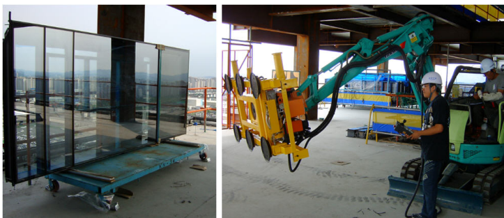
Fig. 1. Curtain-wall for skyscraper and developed curtain-wall installation robot system [1]
