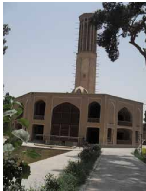
Fig 4. An old house in Yazd with an Air trap
