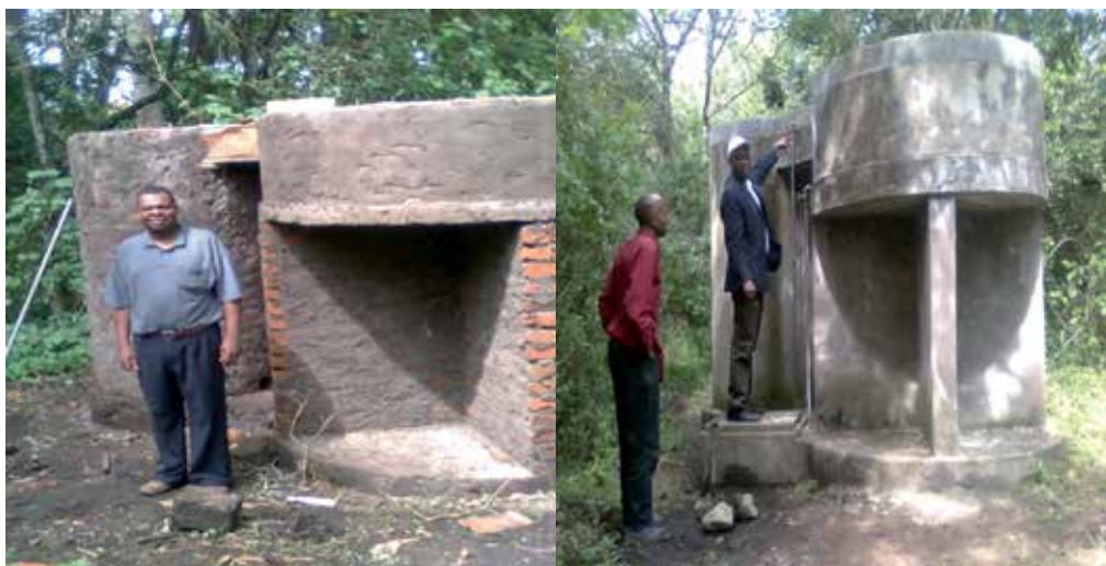
Figure 13. Incomplete and completed community defluoridation unit designed by Ngurdoto Defluoridation research station
