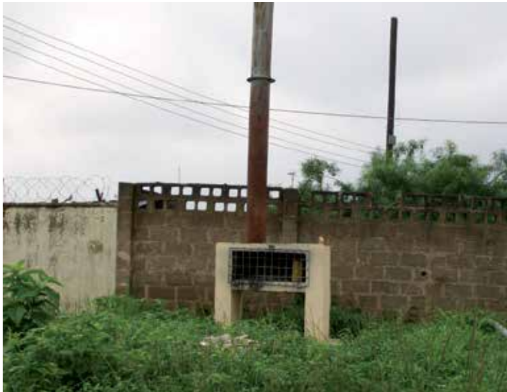
Figure 1. Locally developed incinerator using concrete
