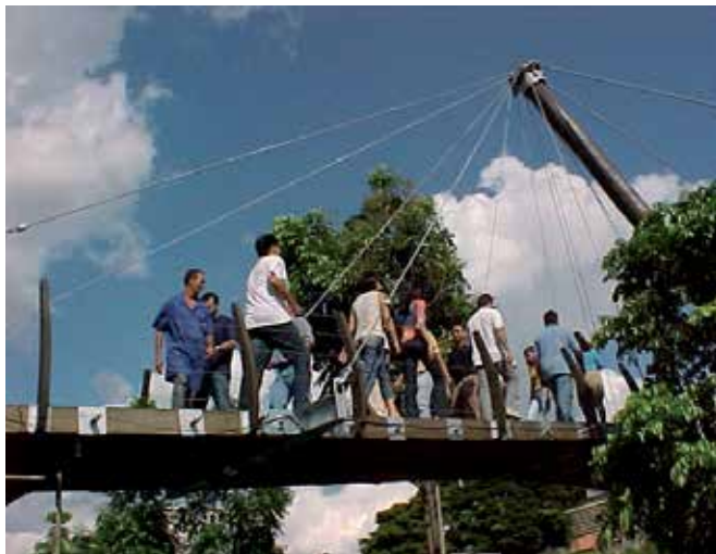
Figure 16. Side view of pedestrians walking over a footbridge
