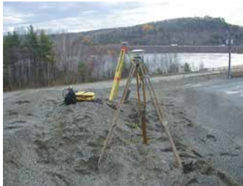
Figure 26. Detail of reference stations used for monitoring the bridge
