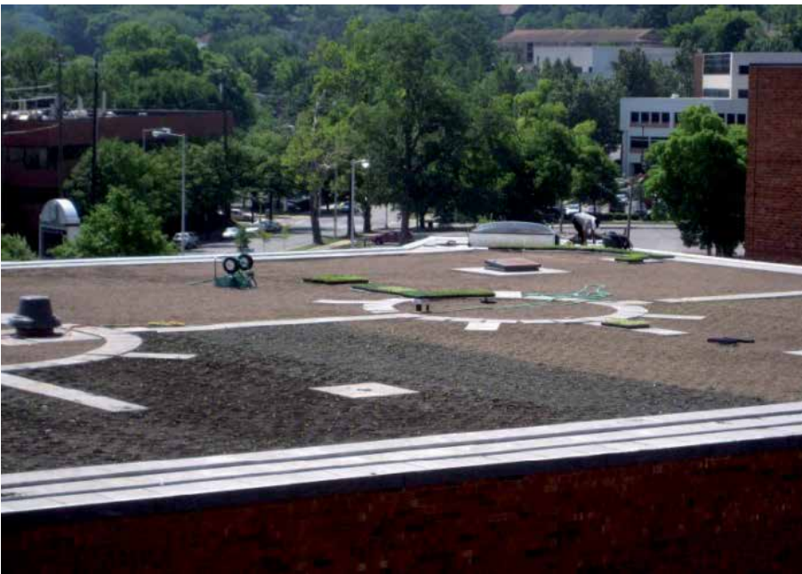
Figure 13. Construction phase for installing a pilot vegetative roof on top of Hulsey Center.
