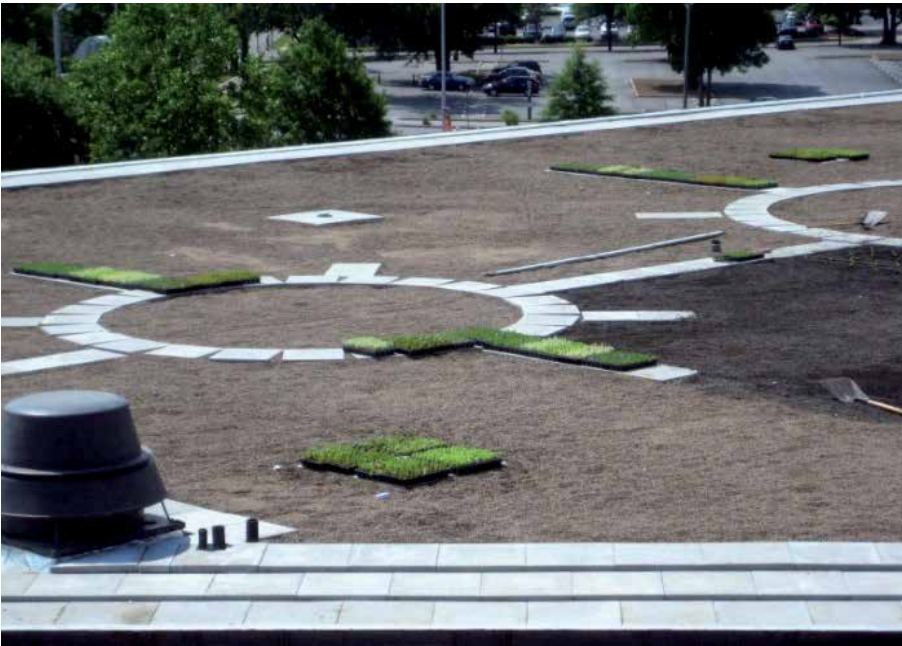
Figure 12. Construction phase for installing a pilot vegetative roof on top of Hulsey Center.
