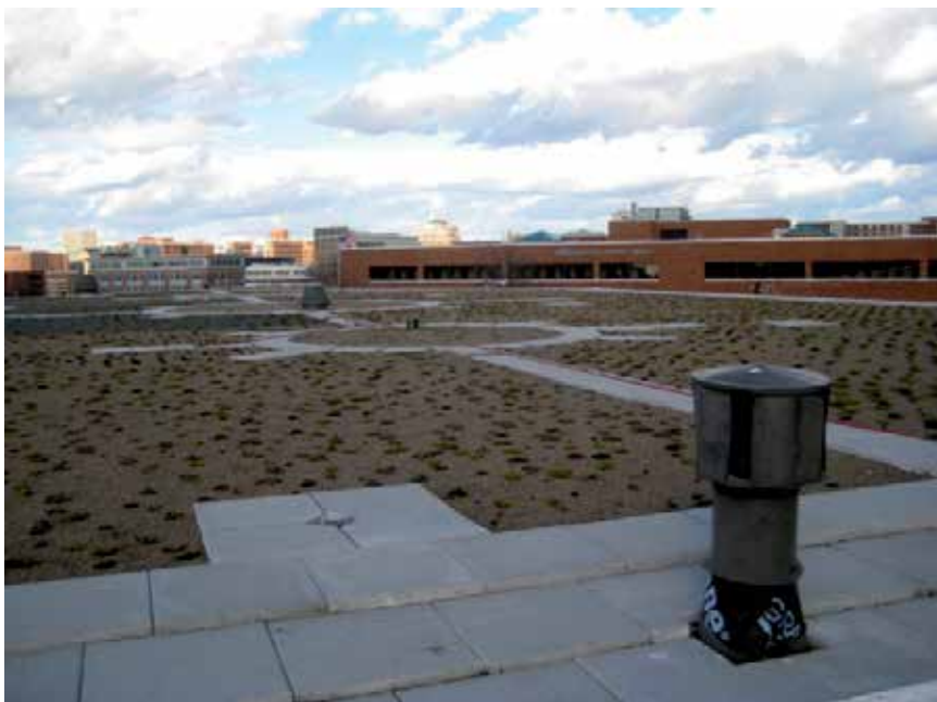
Figure 14. Initial vegetative roof immediately after installation on top of Hulsey Center.
