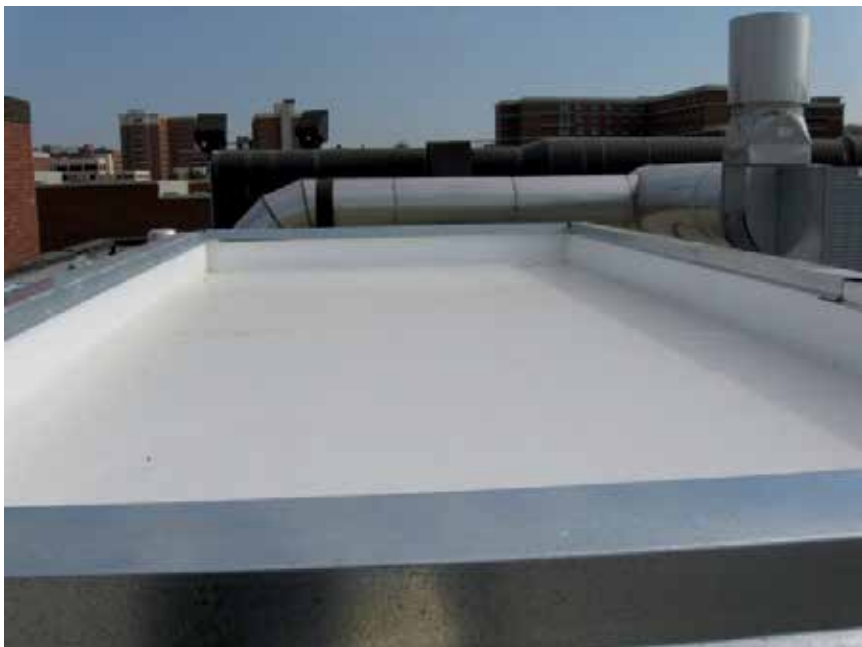
Figure 6. White (reflective) mini-roof.
