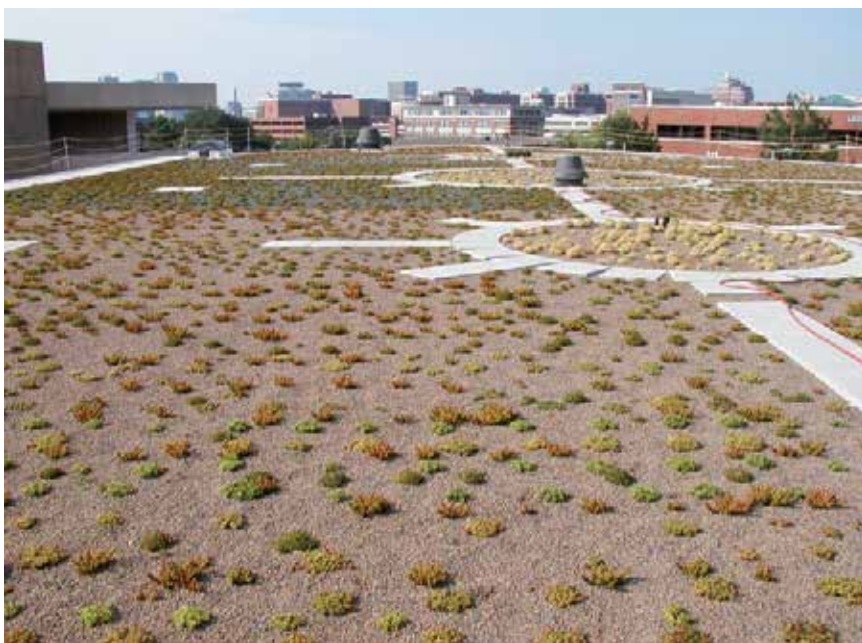
Figure 15. Vegetative roof on top of Hulsey Center (June 2009).
