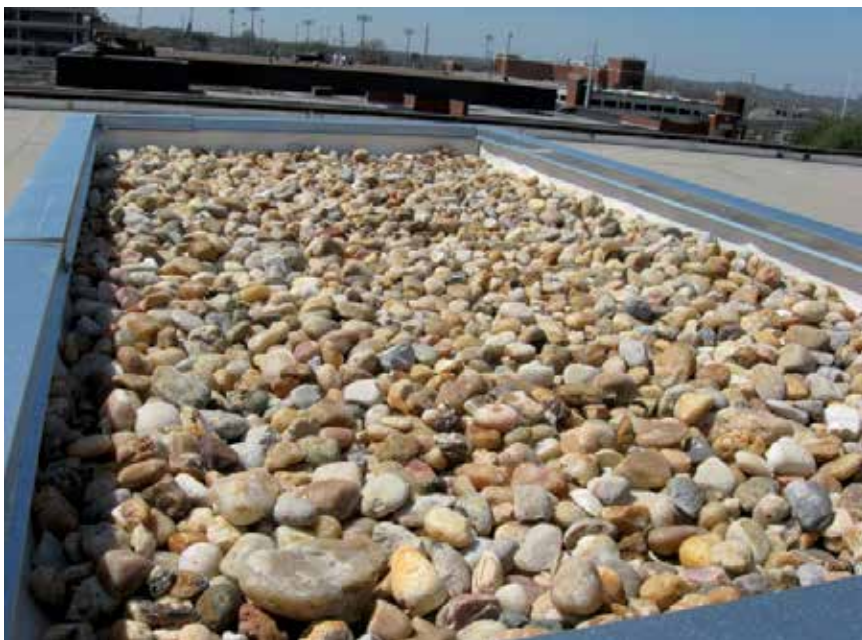
Figure 7. Mini-roof equipped with river rocks.
