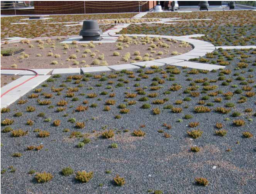
Figure 16. Vegetative roof on top of Hulsey Center (June 2009).
