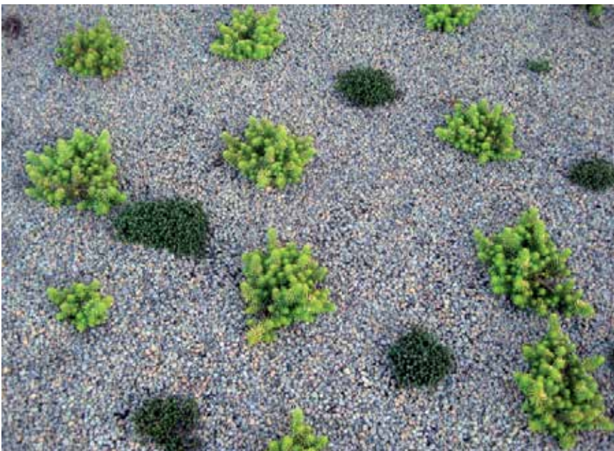
Figure 17. Close-up of vegetative roof on top of Hulsey Center (June 2009).
